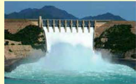
Tarbella Dam Hydro Power 3rd Ext.
